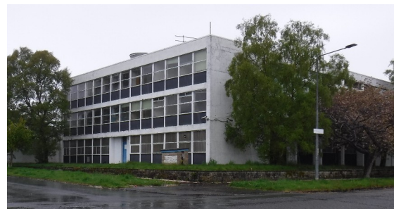
The automatic telephone exchange
